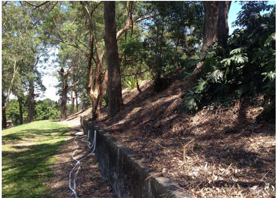
Figure 4.7 The low retaining wall at the toe of the batter below the bowling greens.
